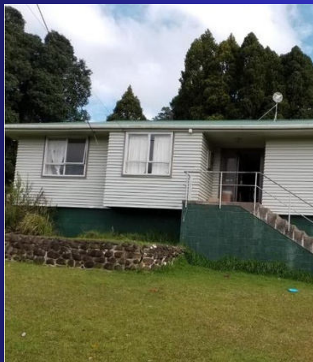
House Upgrade Project
