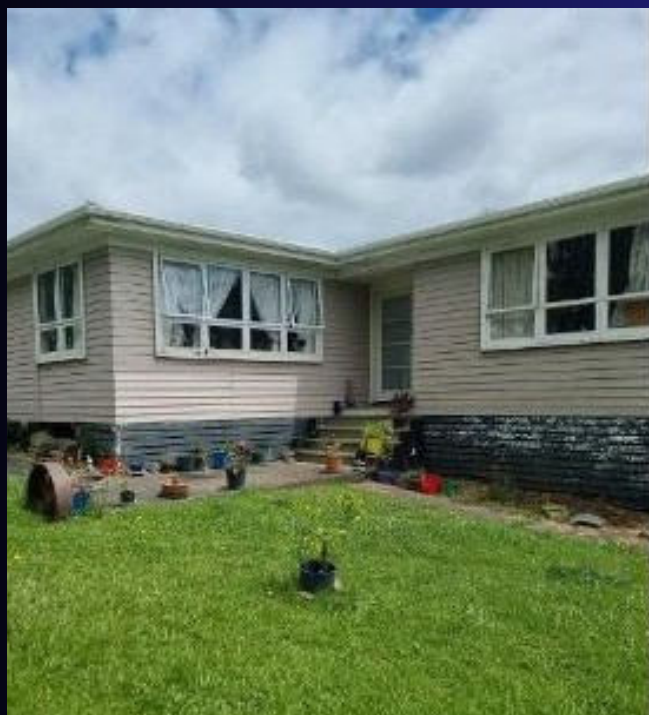
House Upgrade Project
